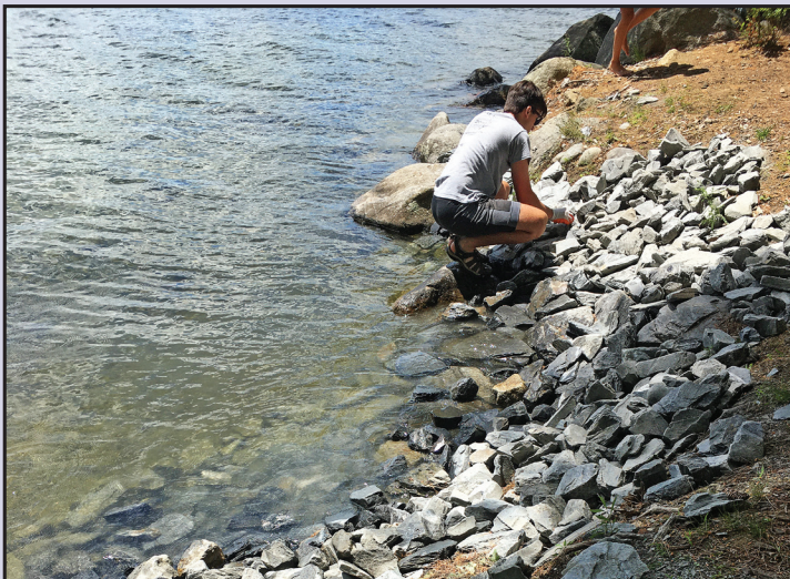
Brennan Dunton is installing riprap (expertly).
